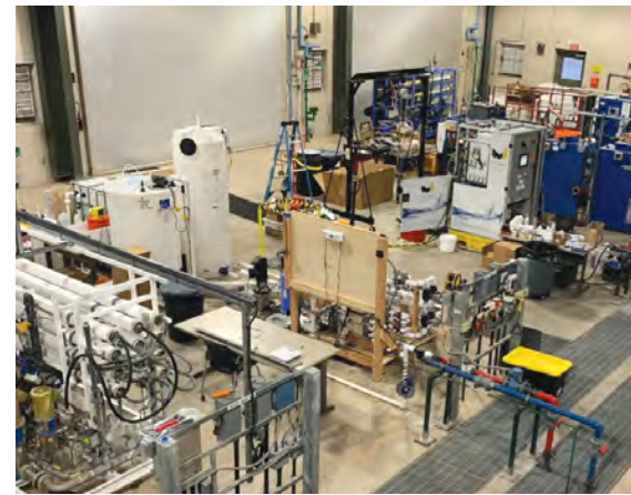
FIGURE 1. BGNDRF Engineering Bay. The 4-inch RO test skid where pilot was performed is in front.
